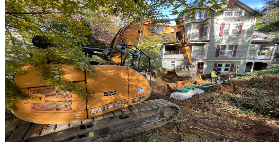
Example of I/A septic system being installed in Sea Cliff.
